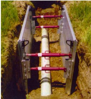
Support systems, shield systems, and other similar protective systems include timber shoring, aluminum hydraulic shoring, and others approved by a registered professional engineer. The top edge of the shielding must protrude 18 inches above the trench.
